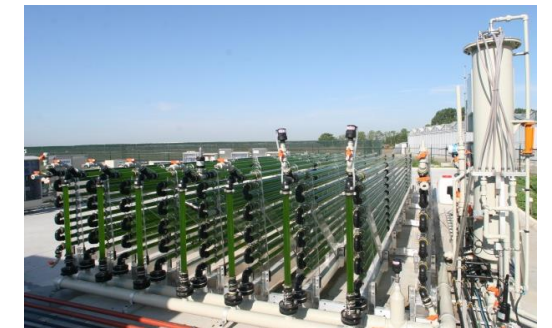
Horizontal tubular PBR 0.56 m 3
